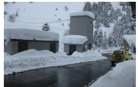
Bielsa tunnel (Spain-France)
